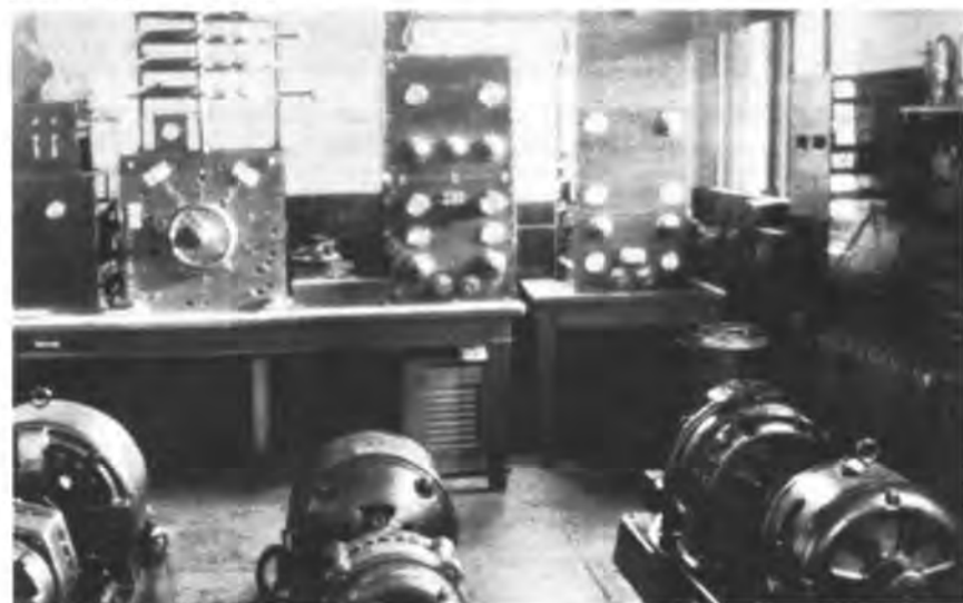
"NAJ" - GREAT LAKES - U.S. NAVY - 1930 E.A. "Art Peavy - 1507-V [WSUZV] contributed this bit of nostalgia. LF at left was a composite rig built from 'left over' spark parts. Work mostly by Ralph Mathew and Fred Schnell (Lts. in USN). Art says a pile of bolts like these old rigs today would put the modern young 'op' in a straight jacket before end of his watch ! Never thought of a 'break-in' with those noisy generators. A bit of nostalgia from the "Windy City".
